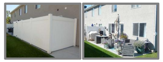
White Vinyl Fencing separates each unit from the adjacent neighbor. Fence is in good condition with minimal signs of wear and tear at the time of our review. Local vendor has indicated the fence shouldn't need replacement for an extended period of time, only repair of damages incurred from lawn mowing, children playing, etc. should be necessary. We
