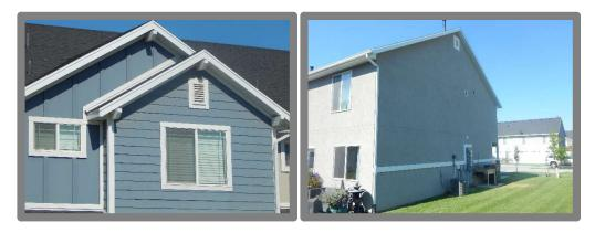
The siding was in good repair for the age of the complex as of the day of our review. Siding for these units is hardy board and stucco and will need periodic repair as it
