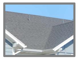
Roof is 30 yr architectural shingles which show no visible signs of wear. They are in good condition and there are no signs of damage throughout the property. Recommend full replacement after approximately 27 years along with gutters and downspouts to take advantage of economies and ensure proper long term functionality.
