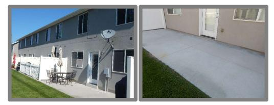
Concrete porches and patio areas on the property were generally in good shape as of the date of our review. The replacement of the concrete will be a major repair and the expected useful life would be typical for the conditions of this area. Recommend a sytematic process of replacement every 3 years as the concrete ages and loses its integrity. This estimate may need to be revised as wear and tear is monitored in the coming years.
