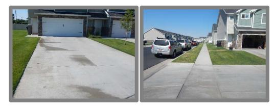
Concrete sidewalks and driveways on the property were generally in good shape as of the date of our review. The replacement of the concrete will be a major repair and the expected useful life would be typical for the conditions of this area. Recommend a systematic process of replacement every 3 years until the property has been restored to its original state of repair. This estimate may need to be revised as wear and tear is monitored in the coming years.
