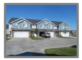
Concrete driveways on the property were generally in good shape as of the date of our review. The replacement of the concrete will be a major repair and the expected useful life would be typical for the conditions of this area. Recommend a systematic process of replacement every 3 years until the property has been restored to its original state of repair. This estimate may need to be revised as wear and tear is monitored in the coming years.
